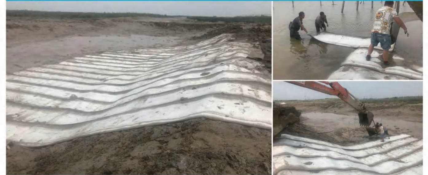
Jiangsu Yancheng Dongtai Luneng revetment project
