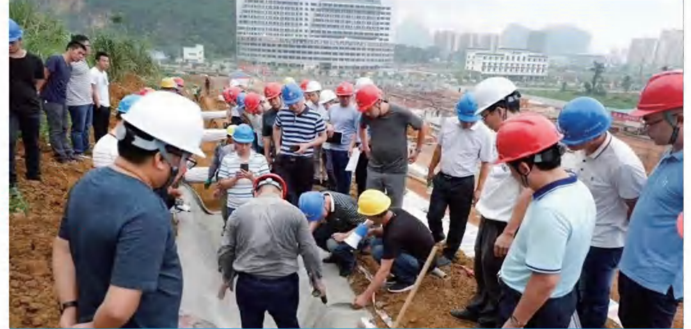
Construction site training meeting
