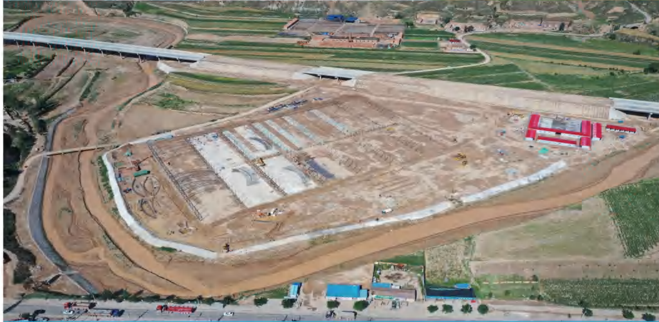
Mineral washing pool
